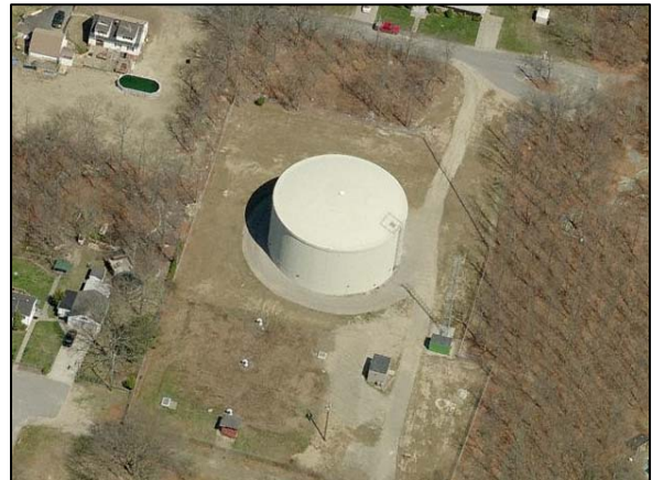
1,000,000-gallon storage tank in Tiverton, RI
